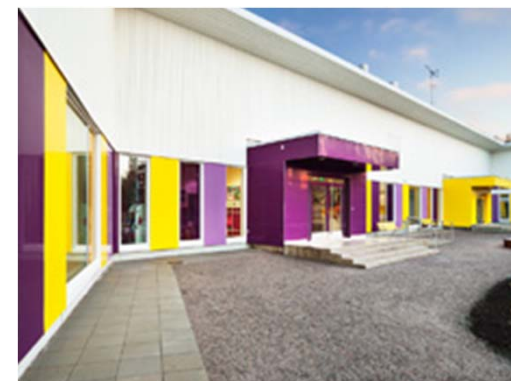
Energy-efficient childcare centre with PPP contract
